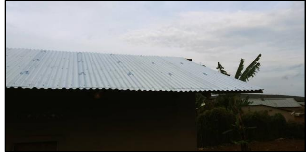
The finished roof.
